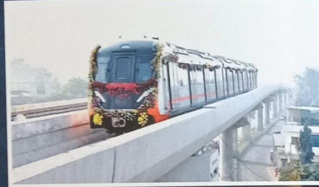
Metro Project - Navi Mumbai
